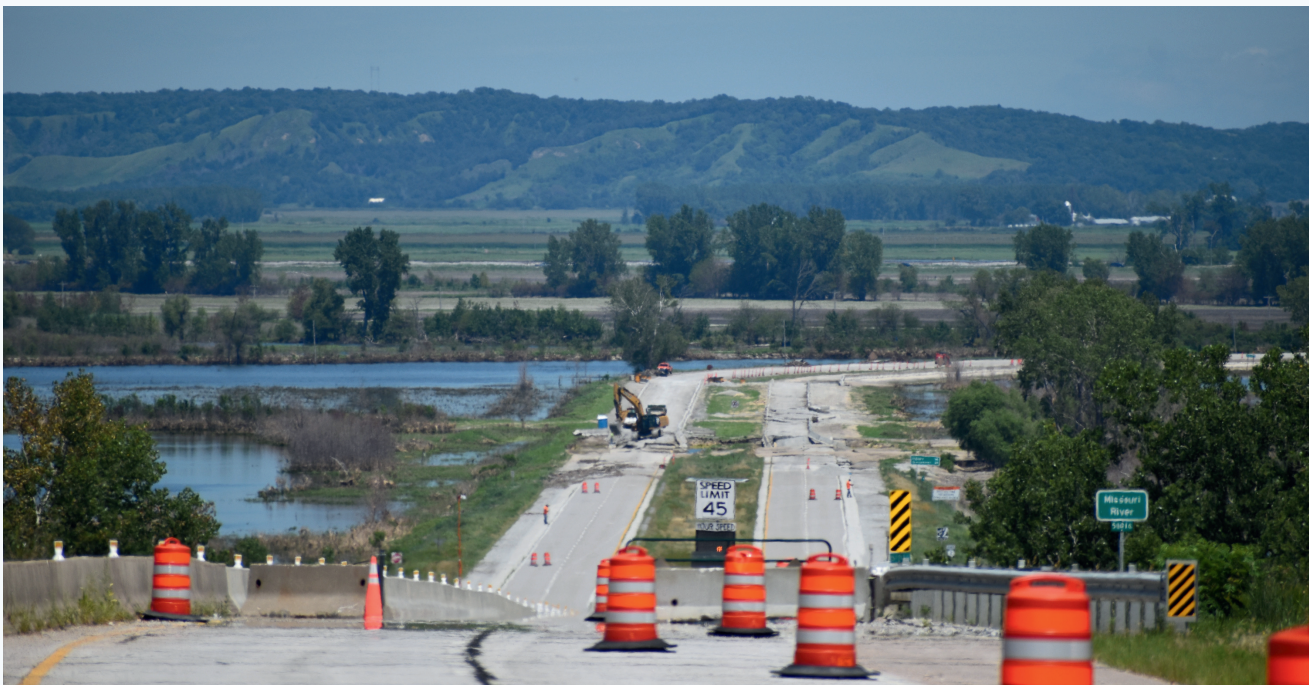
Photo taken by SENDD employee of Nebraska City bridge construction
